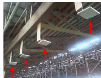
Figure 7. Sirit Infinity 510 circular polarized reader – four antennas at 10 feet.
