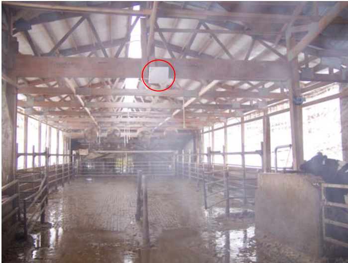
Figure 1. Dairy barn 19 foot alleyway with one fixed reader/antenna attached to a 12 foot beam overhead.
